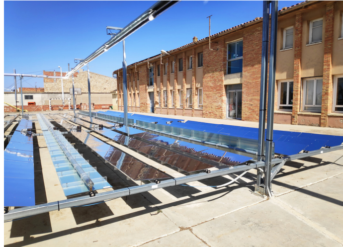
Figure 2. Fresnel solar field and youth hostel building.
