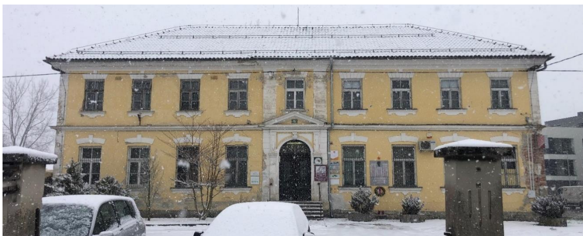
Figure 1. Old school in Ljubljana prior to renovation.
