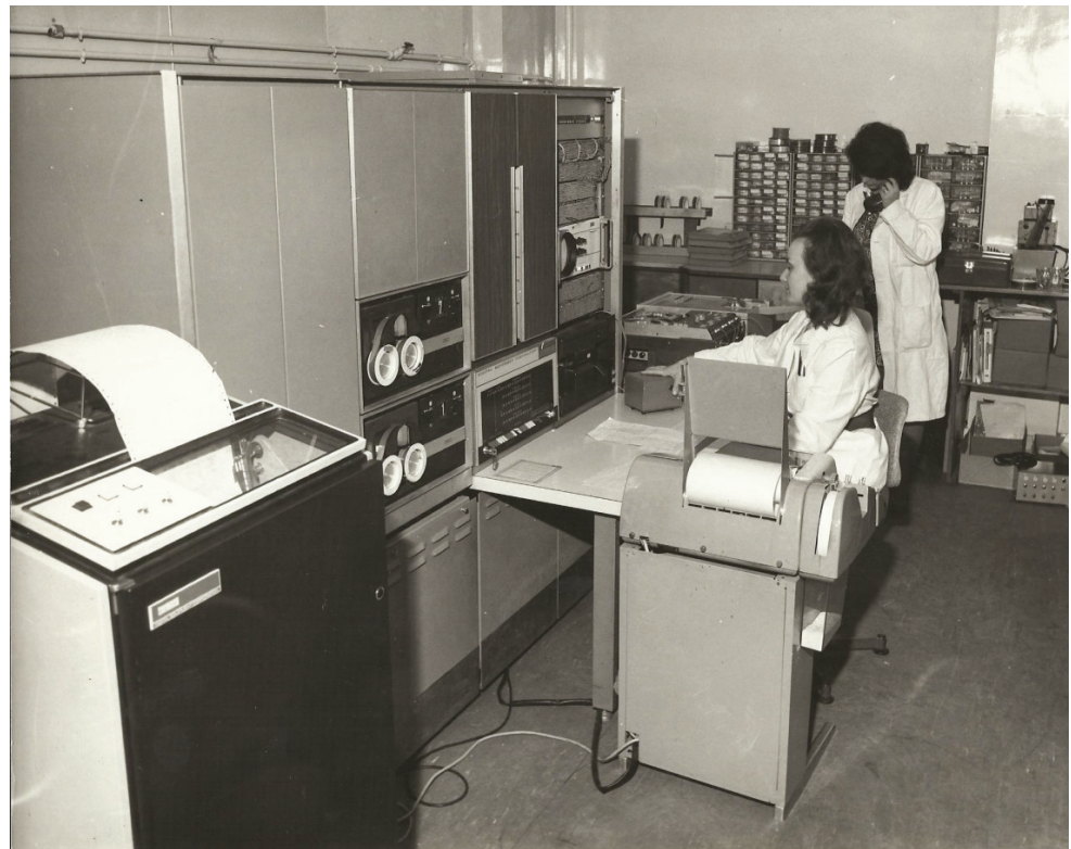
Figure 2. The first automated ECG interpretation system in operation in Glasgow Royal Infirmary around 1971. One technician controlled the tape recorder and listened to the patient details which were also recorded. The second technician monitored the three orthogonal lead ECG on the oscilloscope and started the analogue to digital conversion. The software was stored on the small digital tapes (DECTapes) and retrieved as necessary.
