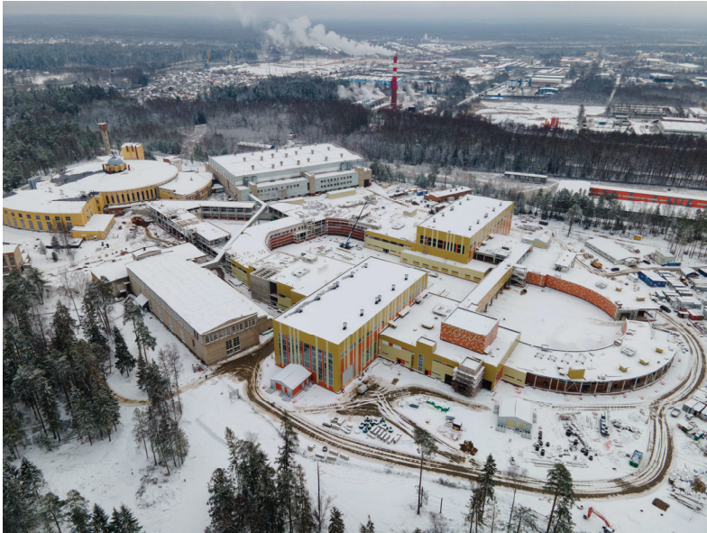
Figure 2: Aerial view of the NICA accelerator complex as of December 2020. The oval ring in front is the collider for protons and nuclei with two interaction points for the MPD and SPD experiments to be hosted in the rectangular buildings. In the back to the left is the synchrotron building which hosts the nuclotron superconducting accelerator serving as the injector to the collider ring, together with the ion source, linear accelerator and booster systems. The adjacent rectangular building is the fixed target hall where the baryonic matter at nuclotron (BM @ N) experiment is located.
