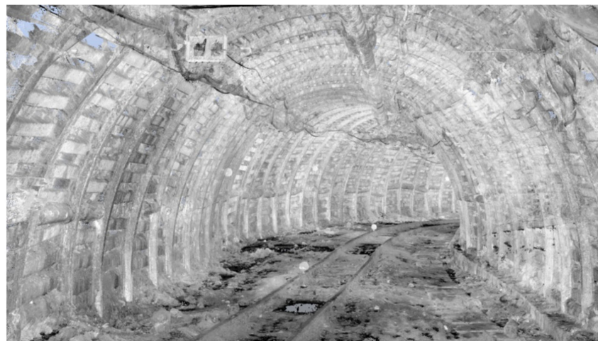
Figure 2. 'Inside' view of a mine gallery section before a bend—point cloud.
