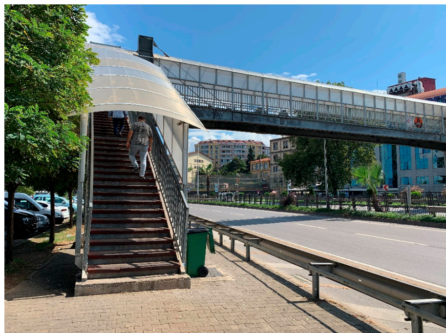
Figure 8. The overpass suspended over the highway no. D010 after constructing the roofing.
