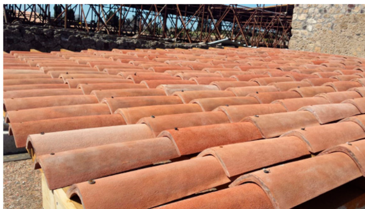
Figure 11. Installation of new Tegola photovoltaic tiles.
