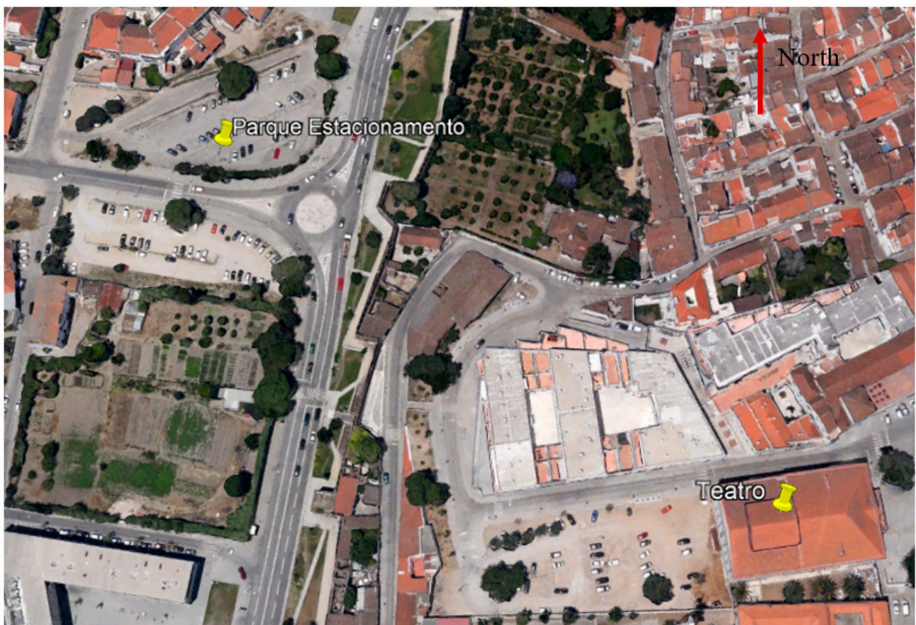
Figure 25. Location of the car park targeted by BIPV solutions on Avenida Engenheiro Arantes e Oliveira, in the vicinity of the Garcia de Resende Theatre.
