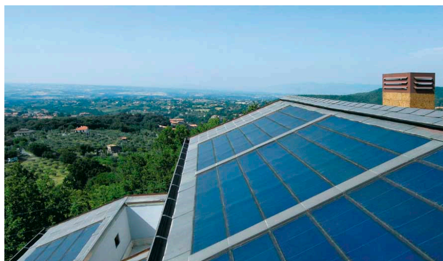
Figure 14. Example of an installation with Tegosolar PV technology.
