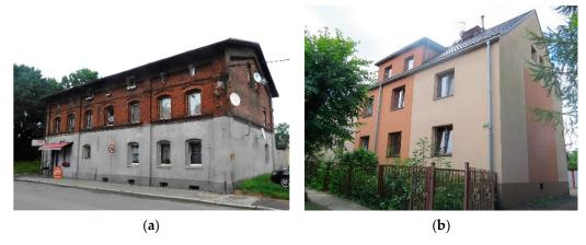
**Figure 4.** Two examples of the 207 masonry buildings qualified for the study: (a) example of a partially renovated building; (b) example building after full renovation.
