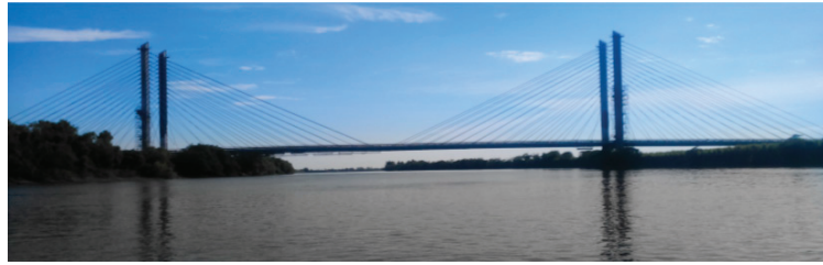
Figure 2. The Rio Papaloapan Bridge.
