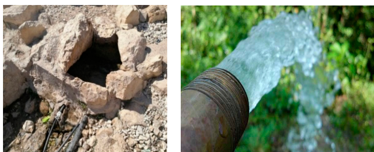
Figure 11. Water borehole in Al-Birin.
