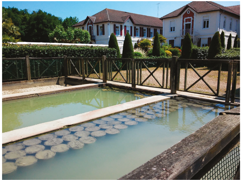
Figure 5. Thermal mud maturation (Dax, France).
