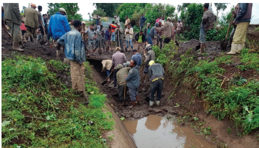
Figure A1. Farmers desilting the sediment from the main canal during the annual desilting campaign at the Ketar irrigation scheme.
