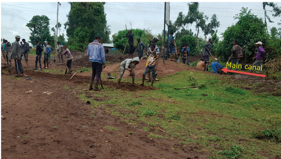
Figure 1. Farmers at the Ketar irrigation scheme diverting surface runoff to prevent sediment from entering the main canal, 25 August 2018.
