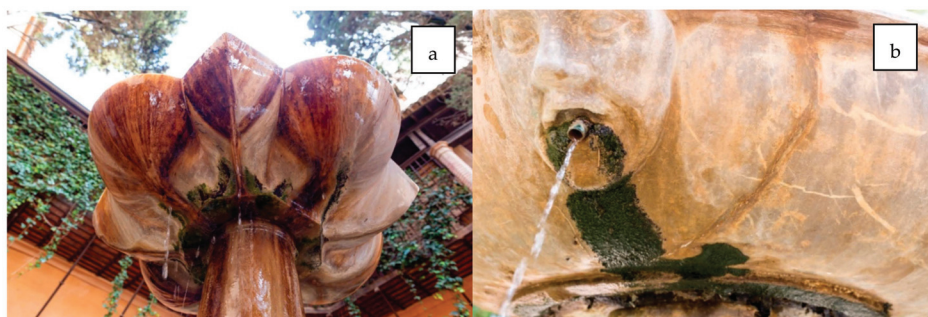
Figure 1. (a) Two different phycofilms on the Fuente del Patio de la Reja at the Nasrid Palaces. (b) Algal mat growing on the Fuente del Patio de la Sultana at Generalife. Photos by G. Alfano.
