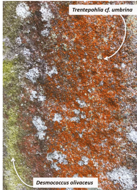
Figure 3. Example of dominance of Trentepohlia cf. umbrina on the N-facing wall of the BAR church.
