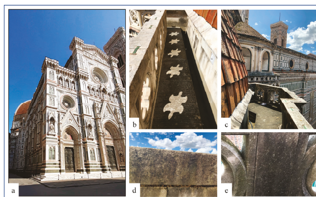
Figure 1. The Cathedral of Santa Maria del Fiore and the study sites. (a) The façade; (b) the external gallery running around the apses of the SE exposed façade; (c) the external gallery on the NW exposed façade; (d) a detail of the marble surface of the inner face of the openwork parapet of the SE exposed gallery; (e) a detail of the openwork parapet at the NW site showing a widespread dark patina.
