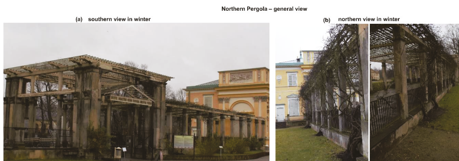
Figure 1. General view of the Northern Pergola in winter from the southern (a) and the north-facing side (b).
