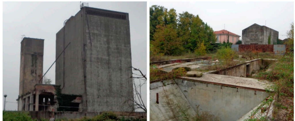
Figure 6. Project area in Inveruno showing the highest of the to-be-demolished existing buildings (on the left) and the existing underground structures (on the right).
