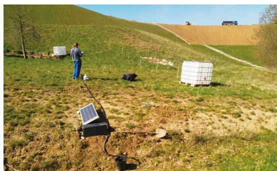
Figure 3. Installation of a solar-powered water pump at plot V2 at the quarry in Ehningen, Southwest Germany during lock-down in April 2020.
