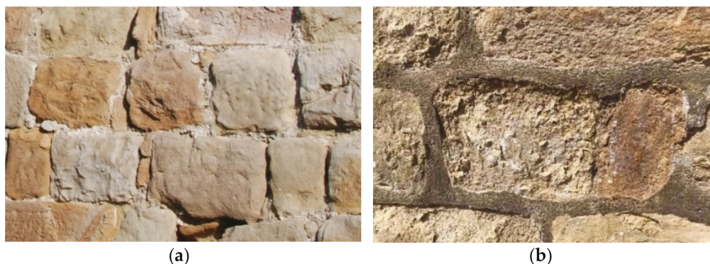
Figure 1. Malpractice of introducing cement-lime mortar in Serbia (a) before July 2012; (b) nine years after repair of the wall—July 2021).
