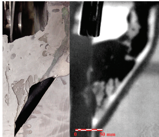
Figure 21. Comparison of NDE findings at the location of the flap lever seating (right) with the actual condition of the adhesive joint (left).
