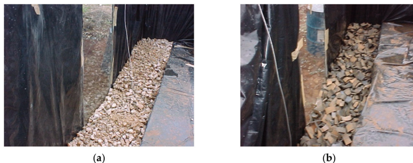
Figure 13. Drainage trenches in containers C1 and C2: (a) C1; (b) C2.
