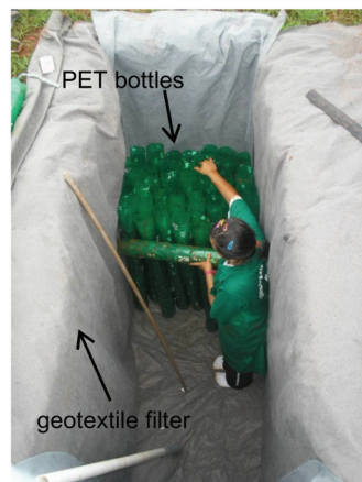
Figure 22. Drainage trench with PET bottles for flood control [82].
