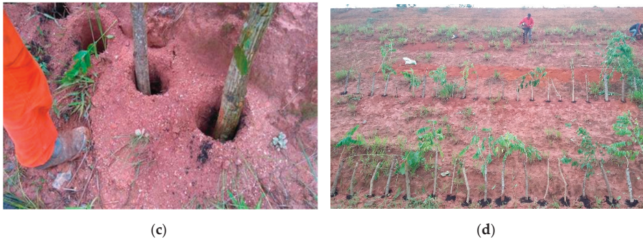
Figure A1. Live stakes: (a) storage after transport in an air-conditioned environment, (b) root system detail, (c) installation procedure in manually excavated cavities, and (d) substrate material application.
