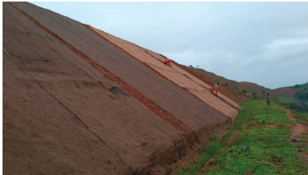
Figure 3. Contiguous execution of the bioengineering techniques with the experimental unit.
