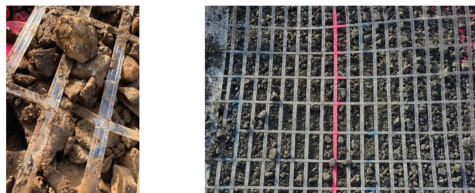
Figure 10. Visual inspection of geogrid after RFID test: left: test with TB; some smaller damages can be seen; right: no damages in tests with BFS, EFS, and RC.
