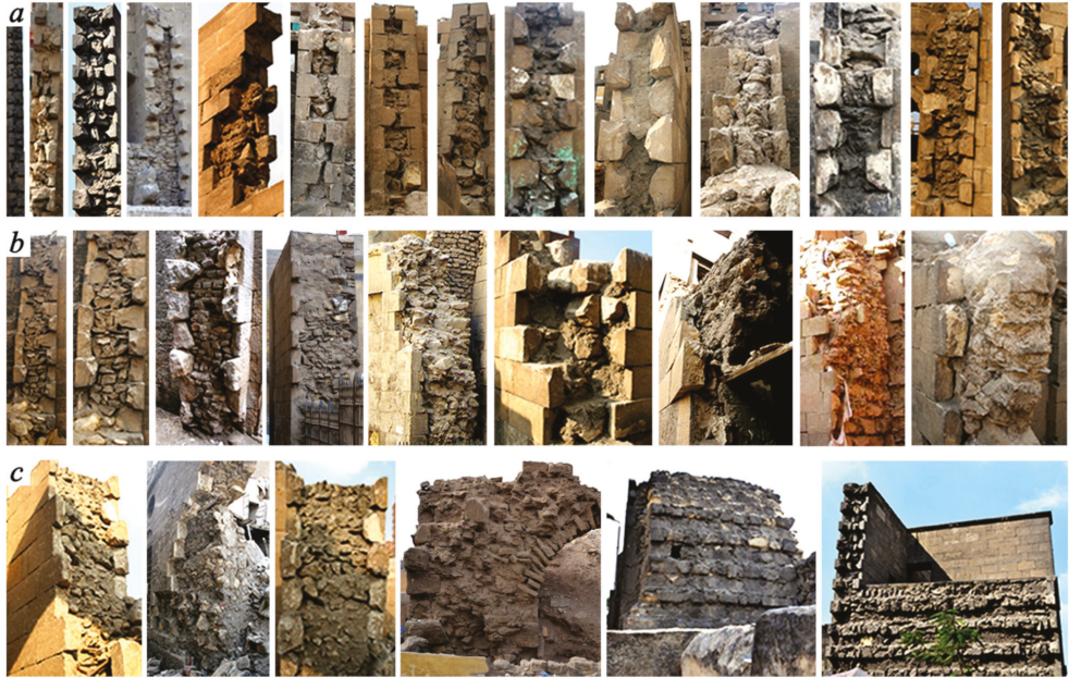
Figure 3. Typical cross-sections of different thicknesses of multiple-leaf stone masonry walls: (a) slender wall [ \frac{Int.}{Ext.} \leq 0.35 ], (b) wall of medium thickness [ 0.35 < \frac{Int.}{Ext.} < 1.5 ], (c) thick (monolithic/massive) wall [ \frac{Int.}{Ext.} \geq 1.5 ].
