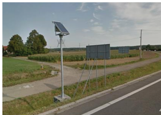
Figure 4. Location of a photovoltaic panel on national road No. 16, distance marker post 38 (Gietrzwałd) (126 + 250 km). Source: [61].
