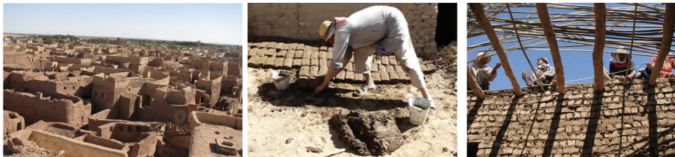
Figure 3. The usage of adobe clay bricks, together with reeds and acacia wood, in construction at Balat Town in Dakhla Oasis.
