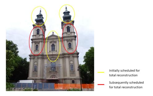
Figure 19. Upper sections of the towers and front façade—proposed total reconstructions.
