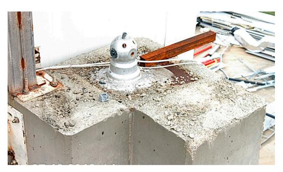
Figure 15. Damage on the support to which the space truss roof system was attached.
