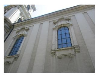
Figure 3. Cracks in the longitudinal wall—north facade.
