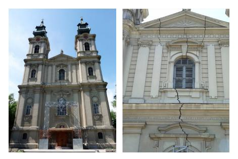
Figure 2. (Left) Cracks in the front facade wall; (Right) Crack details on the upper window.
