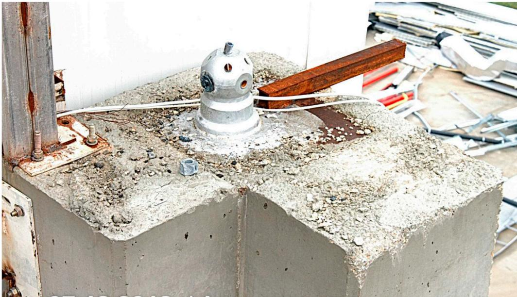
**Figure 15.** Damage on the support to which the space truss roof system was attached.
