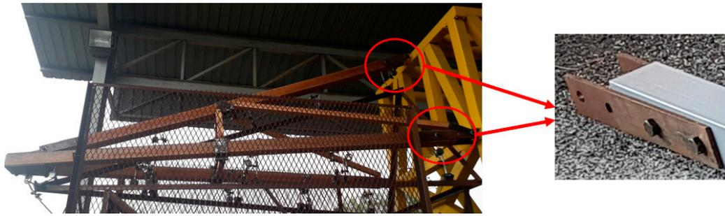
Figure 4. Connection of cross-arm to steel tower using steel plate fittings.
