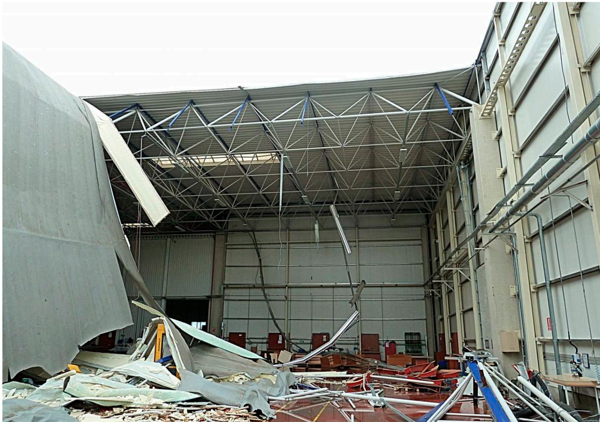
**Figure 4.** Damage to the roof's space truss system.
