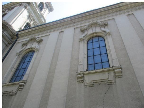
Figure 3. Cracks in the longitudinal wall—north facade.
