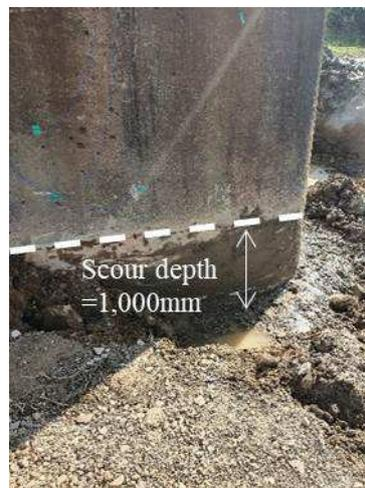
**Figure 5.** Simulated ground scour (scour depth = 1000 mm).
