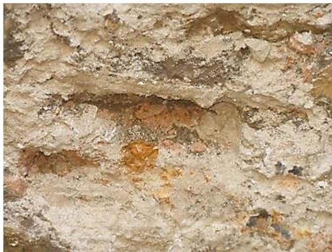
Figure 7. Appearance of the cleaned side surface of the lime concrete foundation.
