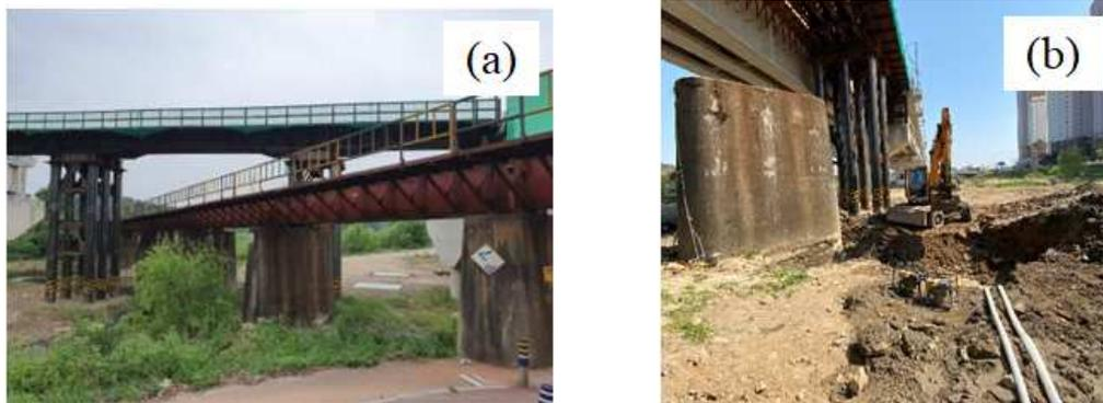
**Figure 4.** Pier of field experiment (a) With girder on the pier and (b) without girder on the pier.
