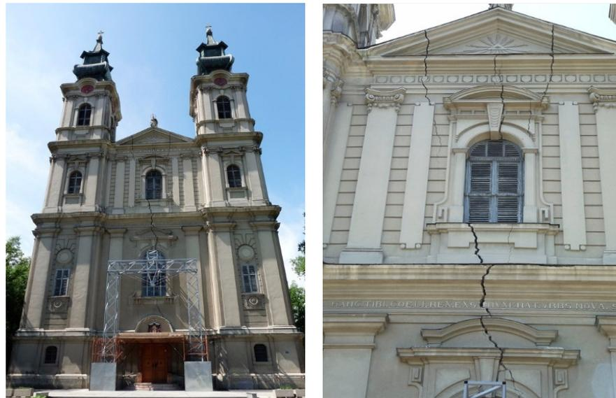
Figure 2. (Left) Cracks in the front facade wall; (Right) Crack details on the upper window.
