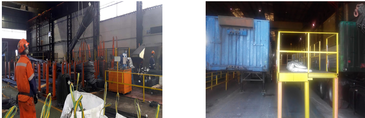
(a) Crane operator at work.
