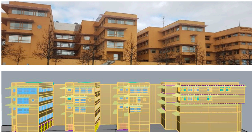
Figure 3. Photo of the real building ( top ) and a 3D render of the building model ( bottom ) showing the south and south-west façades including the permanent overhang. Note that on this side of the building, the basement level is above the ground.
