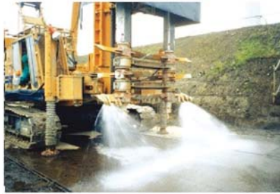
Figure 10. Mixing machine injecting atomized cement slurry [16].
