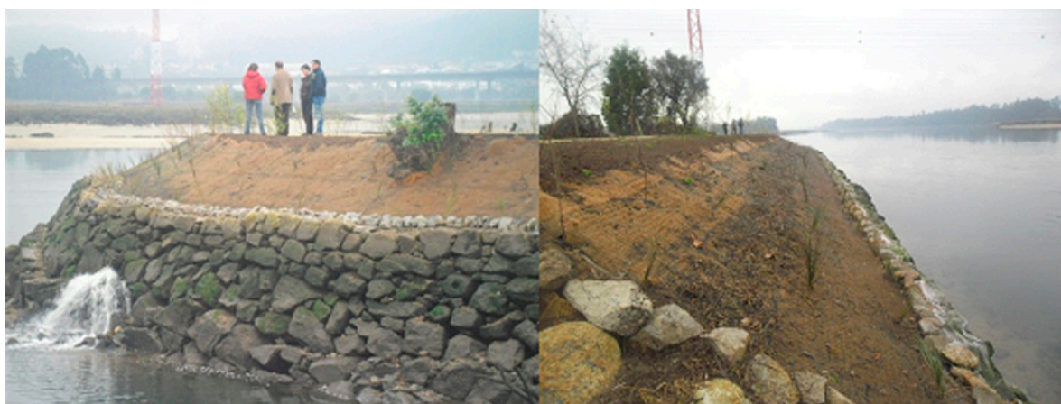
Figure 7. Rip-rap (left) and geogrid disposal (right) in the Portuzelo site (2014).
