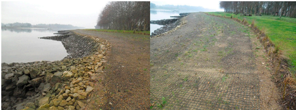
Figure 6. Rip-rap (left) and first row of small groynes (right) in Cardielos, after the implementation of the project in Cardielos in 2014.
