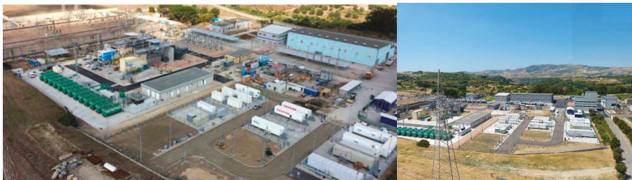
Figure 3. Two views from above the Codrongianos substation.
