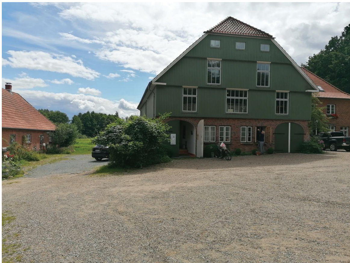
Figure 7. Coworking space in a village, former hayloft, exterior view.
