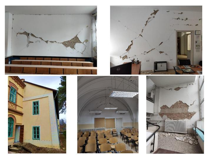
Figure 1. Typical damage to educational buildings after the Zagreb earthquake (photo credit: M. Stepinac).
