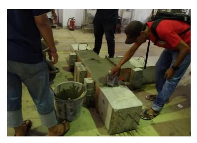
Figure 5. Re-casting the beam-column joint after installing the wire mesh.
