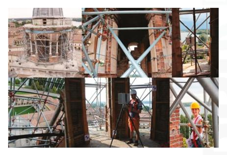
**Figure 5.** Some pictures of survey moments of the "round temple", on the top of the tower. The images shows the difficulties given by the presence of the metal scaffoldings and the wooden holding structure positioned after the earthquake.
