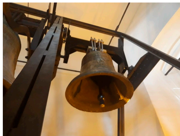
Figure 8. Welded bell attached to the tower.
