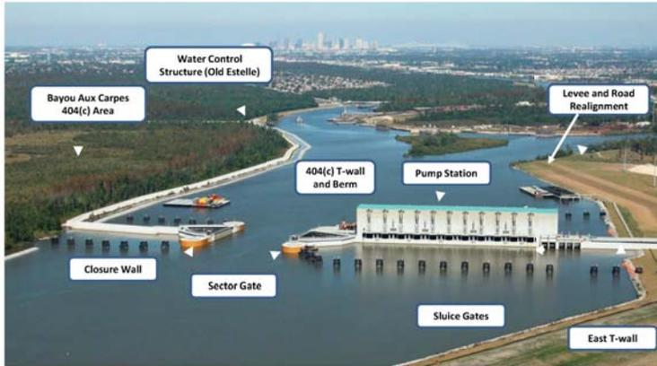
Figure 10. Image of the GIWW—West Closure Pump station.
