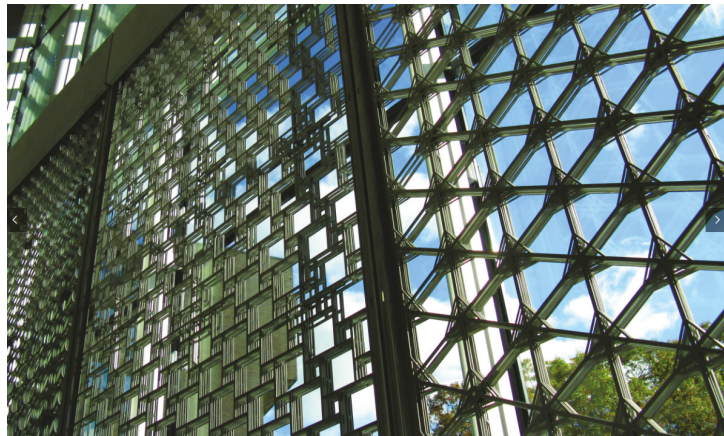
Figure 1. An example of shading devices used as an essential part of a structure for controlling solar radiation is the dynamic windows at the Simon Centre for Geometry and Physics at the State University of New York, USA (2010) (Source: https://www.hoberman.com/portfolio/dynamic-windows/ ).
