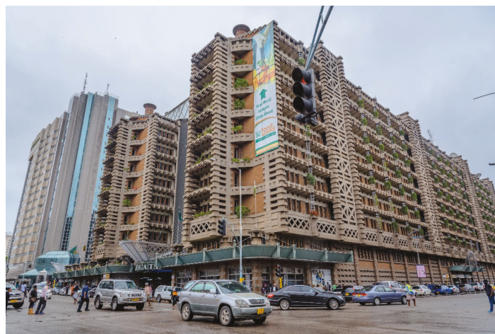
Figure 3. The Eastgate Centre has mimicked termite performance in passive cooling through the use of local material and porous building.
