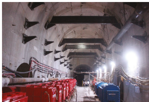
Figure 12. Field effect of pump house after reinforcement.
