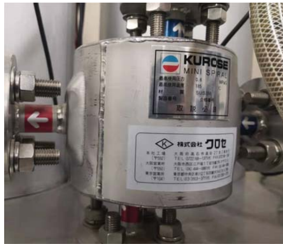
Figure 1. A spiral-plate heat exchanger plant.
