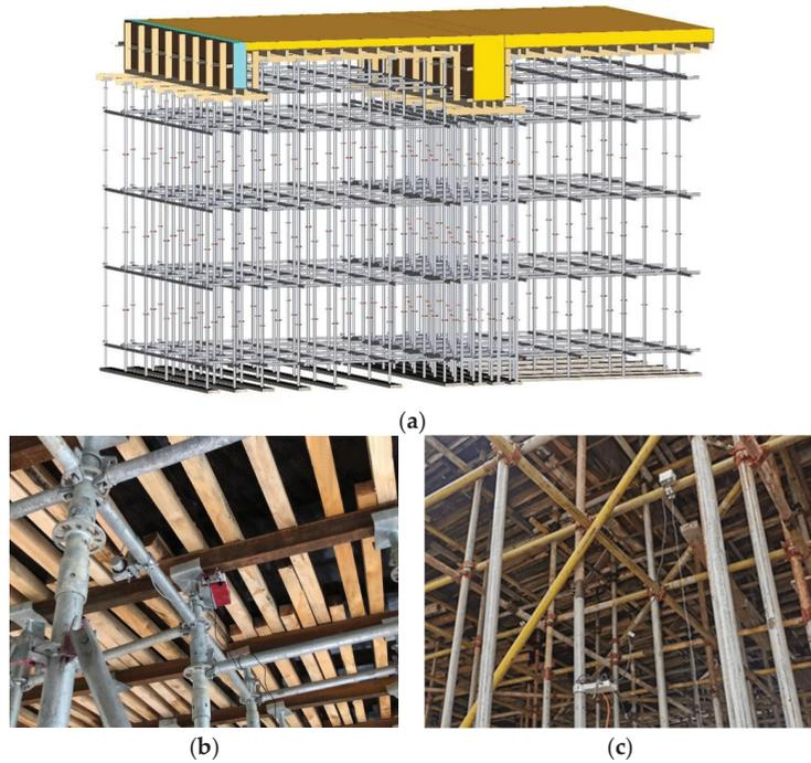
**Figure 11.** Monitoring arrangement of the high formwork system: (a) the 3D model of the high formwork; (b) the installation of the collector; (c) the installation of the analyzer.
