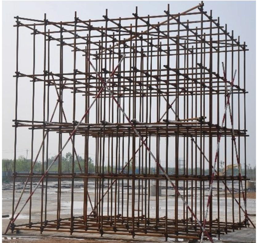
Figure 20. The photography of the high formwork.
