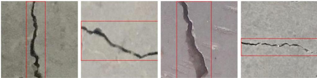
**Figure 9.** Detection results of the concrete surface cracks.
