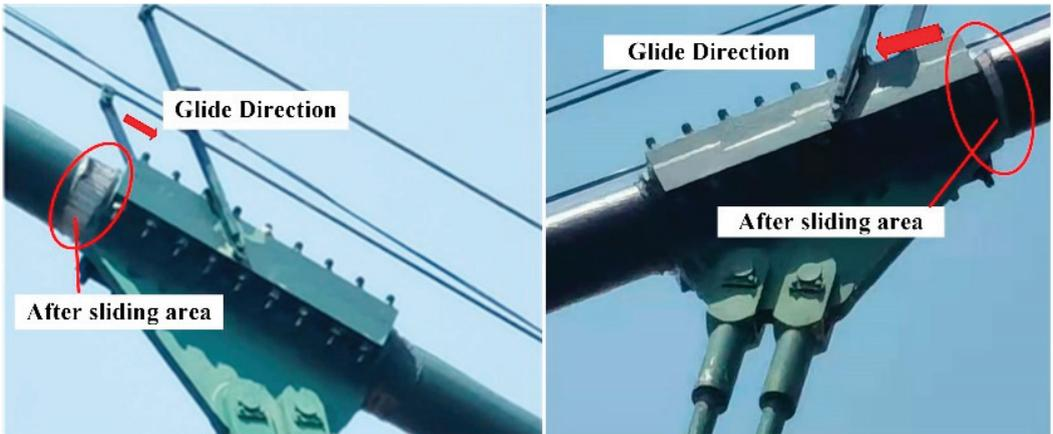
**Figure 2.** Actual images of a cable clip after slipping.
