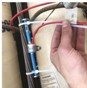
Figure 3. Vibrating wire strain gage placement.
