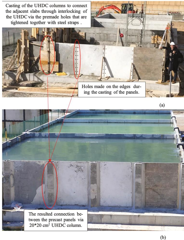
**Figure 2.** Pictures of the structure, taken on 13 February 2020 (a) and on 20 April 2021 when a full load test was performed filling the three basins (b).
