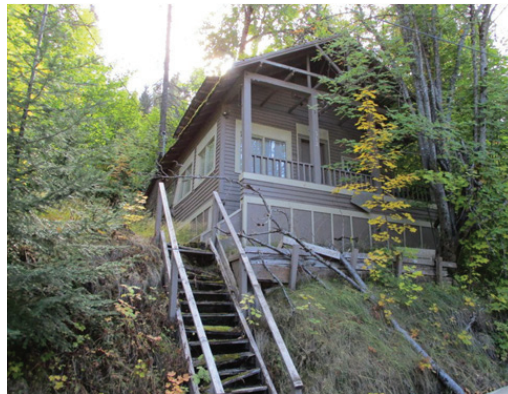
Figure 12. Miner’s cottage in Wallace constructed directly above downtown on terrain too steep for street access.
