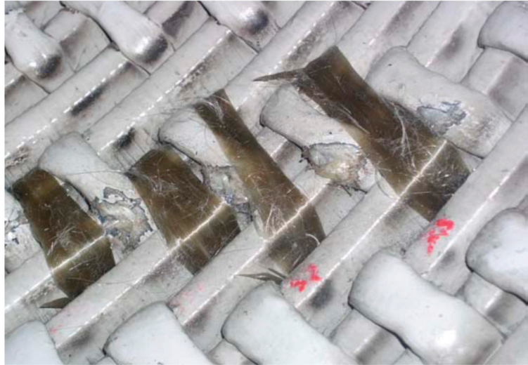
Figure 3. Restored ties with glass roving and resin.
