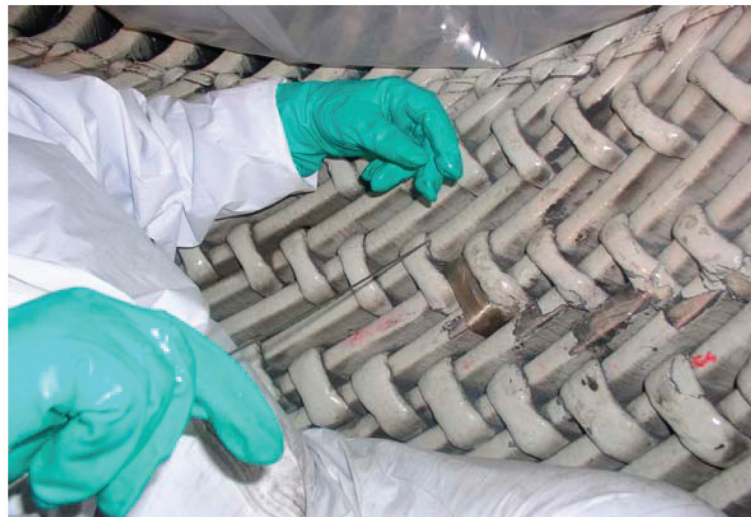
Figure 2. Restating ties with glass roving and resin.
