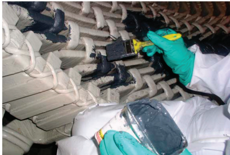
Figure 4. Painting of the restored area with resin.
