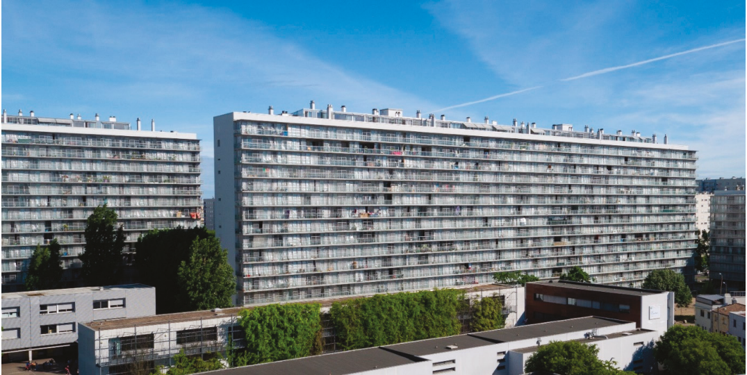
Figure 2. Renovation of a complex of three fifteen-storey blocks in the Grand Parc in Bordeaux. Pritzker Prize 2021. Architects: Anne Lacaton and Jean-Philippe Vassal, adapted from Ref. https://www.pritzkerprize.com/sites/default/files/inline-files/Transformation%20of%20G%2C%20H%2C%20I%20Buildings%201.jpg photo Philippe Ruault, (accessed on 13 May 2022).
