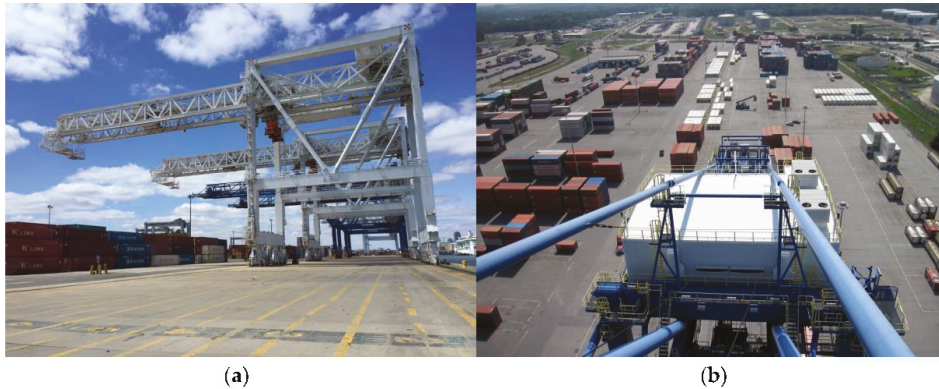
Figure 2. (a) Photograph of the “Apron” area at the Port of Boston; and (b) photograph of primary (to right) and secondary (to left) yards in Wilmington, North Carolina (photos by A. Becker).
