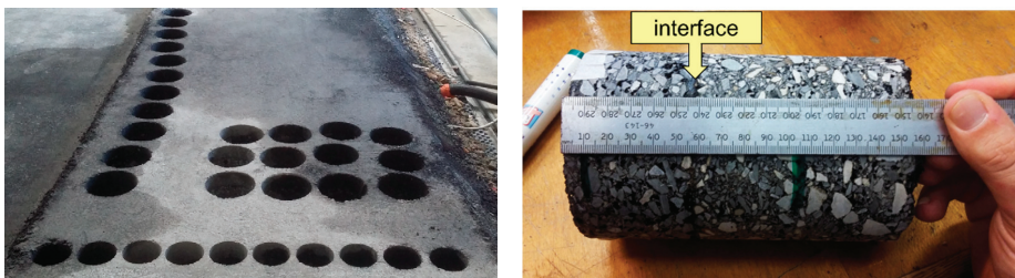
Figure 4. (a) Detail of the trial section after coring; (b) cored specimen.
