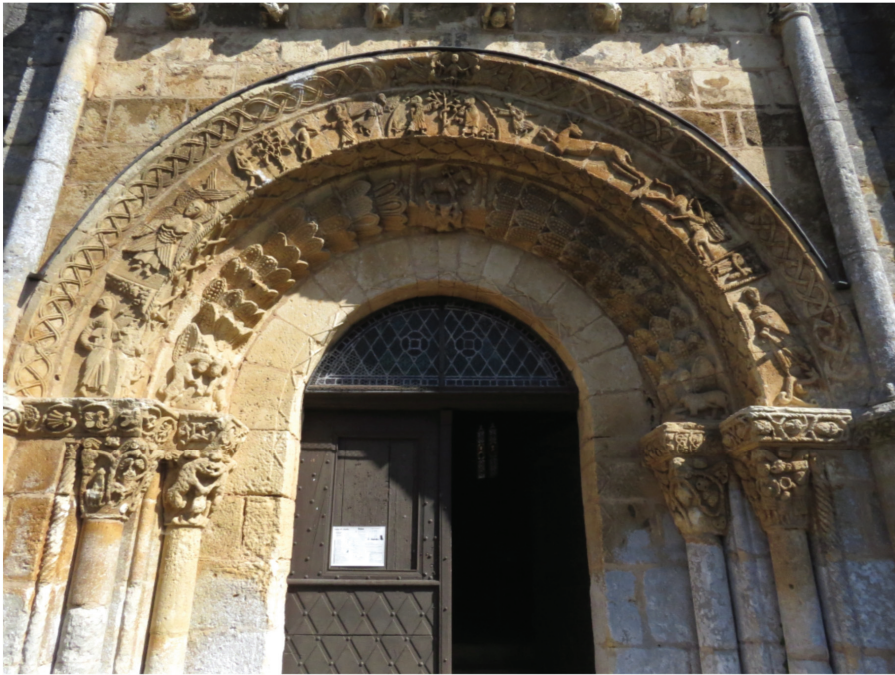
Figure 3. Archivolt, detail of west façade, Saint-Martin Church , 12th c., Besse, Dordogne, Nouvelle-Aquitaine, France. ©Author.
