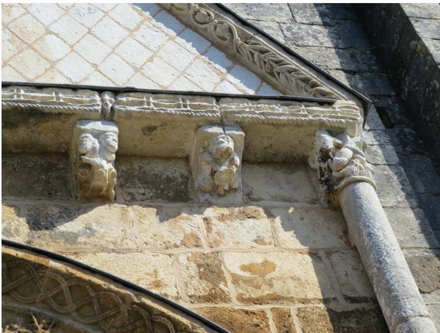
Figure 18. Corbels, detail, west façade, Saint-Martin Church , 12th c., Besse, Dordogne, Nouvelle-Aquitaine, France. ©Author.
