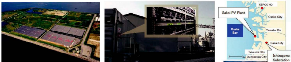
Figure S6. Solar farm and Ni/MH BPS near Osaka, Japan [S7].
