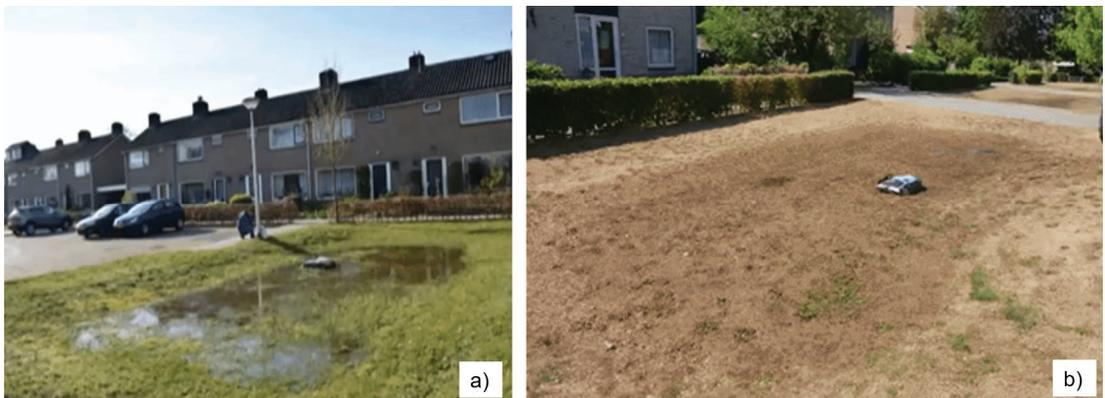
**Figure 1.** (a) Swale at study site in the municipality Dalfsen showing normal condition in 2017 and (b) the same swale after a 7-weeks dry period in 2018. The swales in Dalfsen is the case study presented in this paper.
