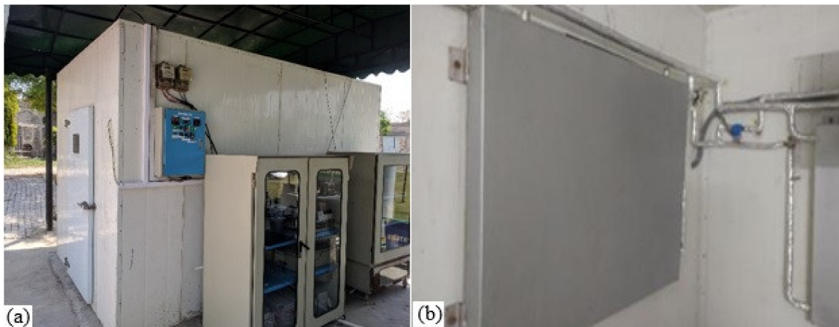
Figure 2. Photographic view of the solar cold storage unit. (a) Cold storage and data monitoring system and (b) inner view of the cold storage and the brine pads.
