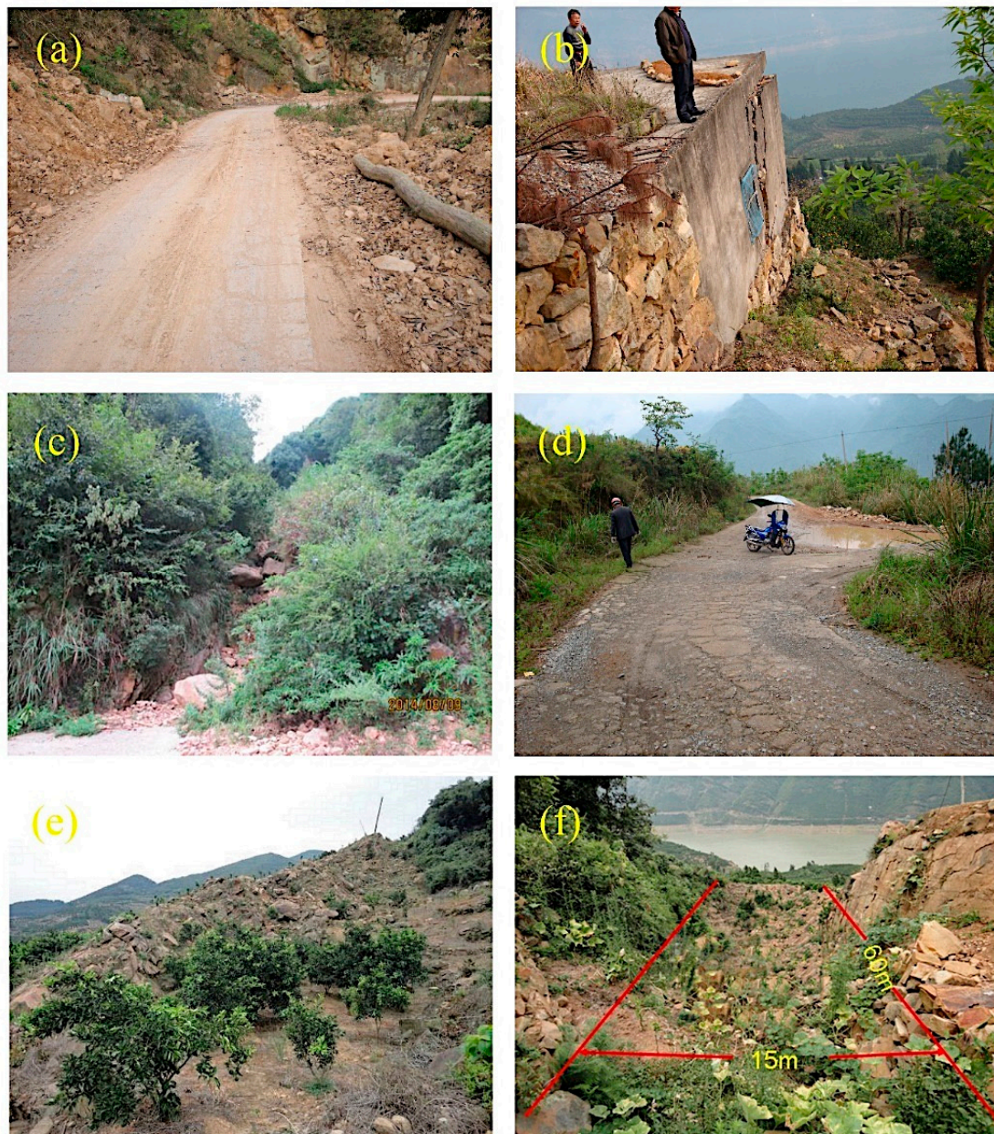
Figure 4. Deformations on the Muyubao landslide: (a) road damage on the west boundary, (b) deformation of buildings, (c) a local collapse on the west side, (d) road damage on the east side, (e) a collapse in the middle of the west side and (f) a tensile trench on the east side.
