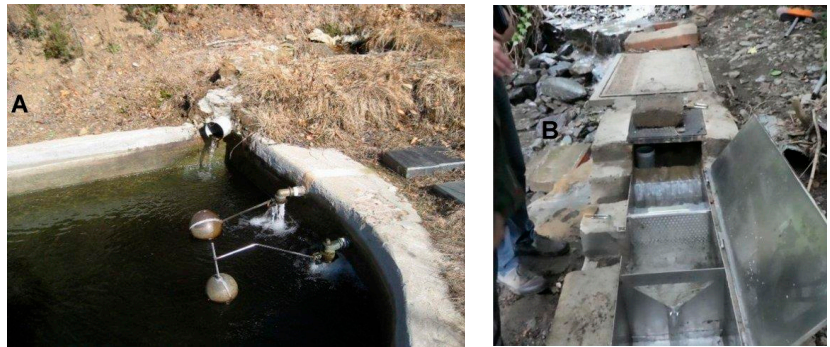
Figure 12. Installed mechanisms which regulate water extraction (A) and distribution boxes (B) restricting the amount of legally allowed water for exploitation.
