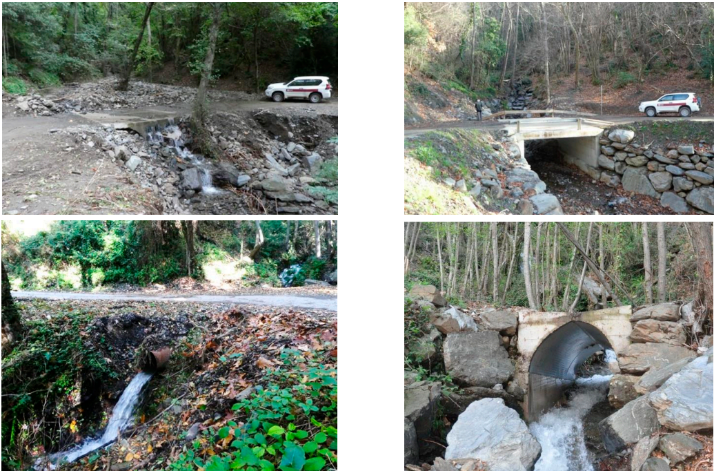
Figure 14. Modified bridges to recover the natural stream bed and to allow the displacement of aquatic fauna along them. Left images: before recovering structure. Right images: the same locality after recovering structure.
